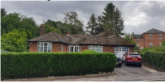
Front elevation with Grade II Listed Building In the background
